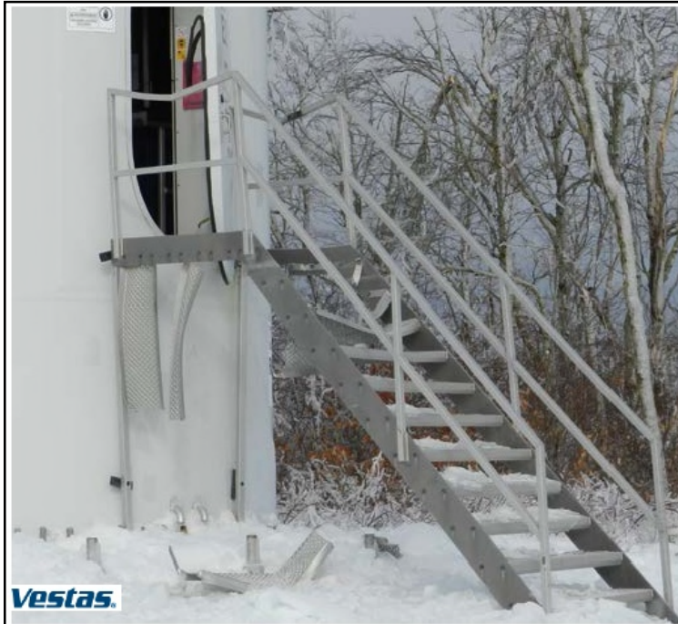
Figure 19: Damaged stairs from an ice fall
