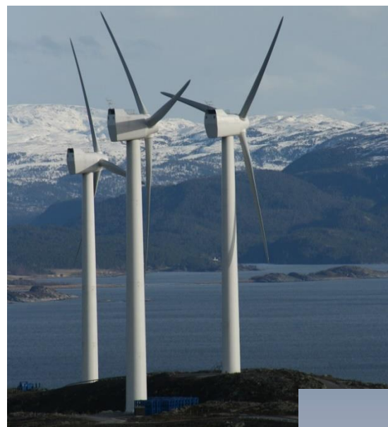
ScanWind SW3.5-90 Diameter 90 m, 3.5 MW
