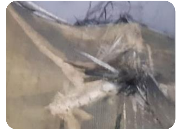
FLASH OVER DAMAGE
