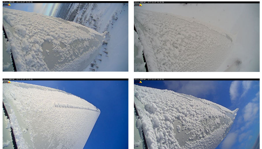
Iced wind turbine blade
