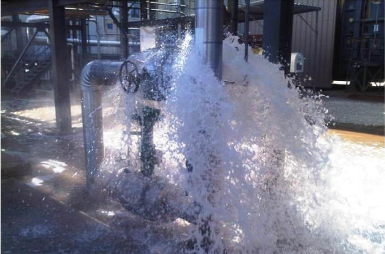
**2011: Frozen valves:** Insulation not re-installed for winter
