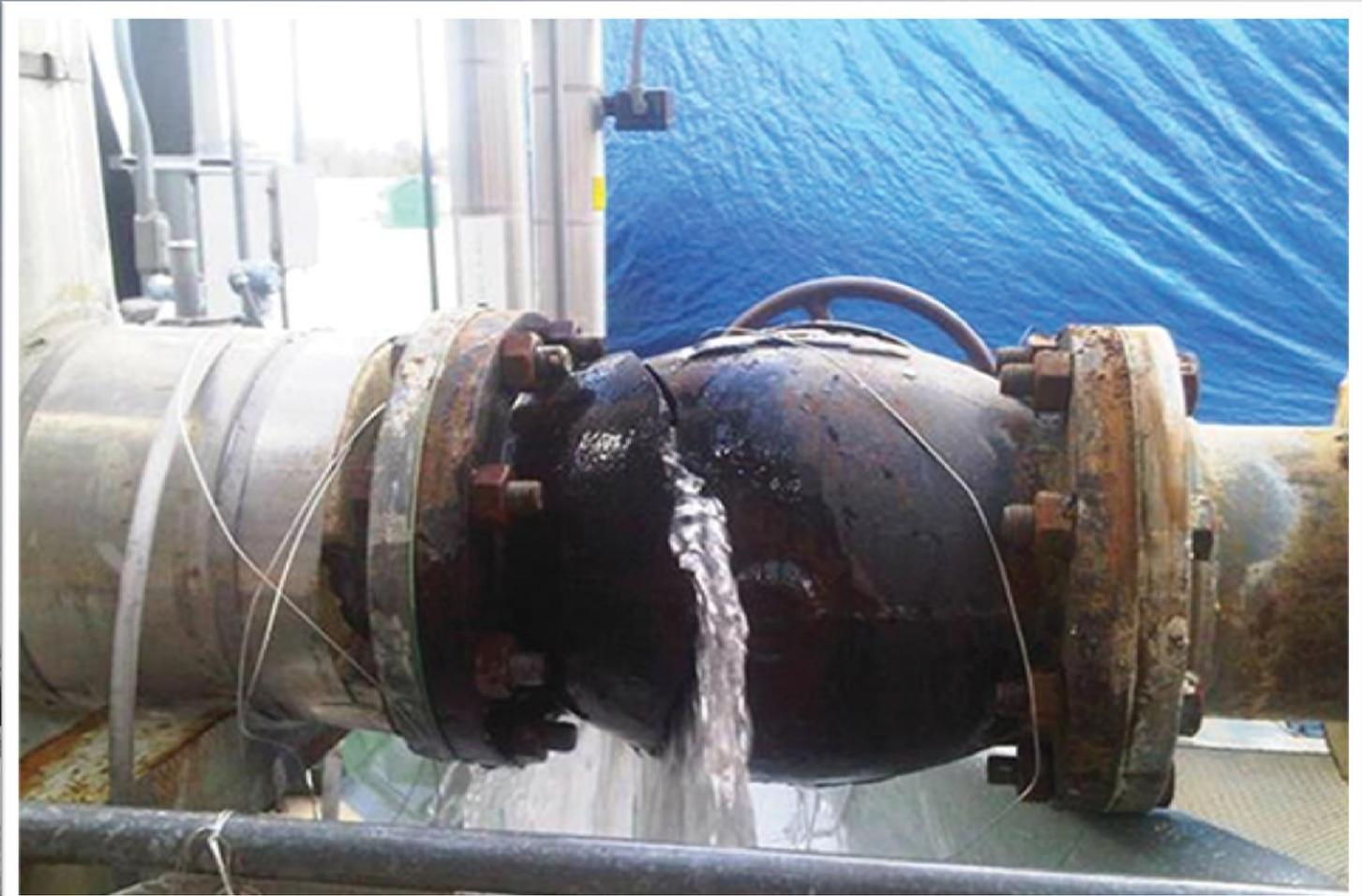
**2011: Frozen pipes:** Frozen water in pipes cause damage
