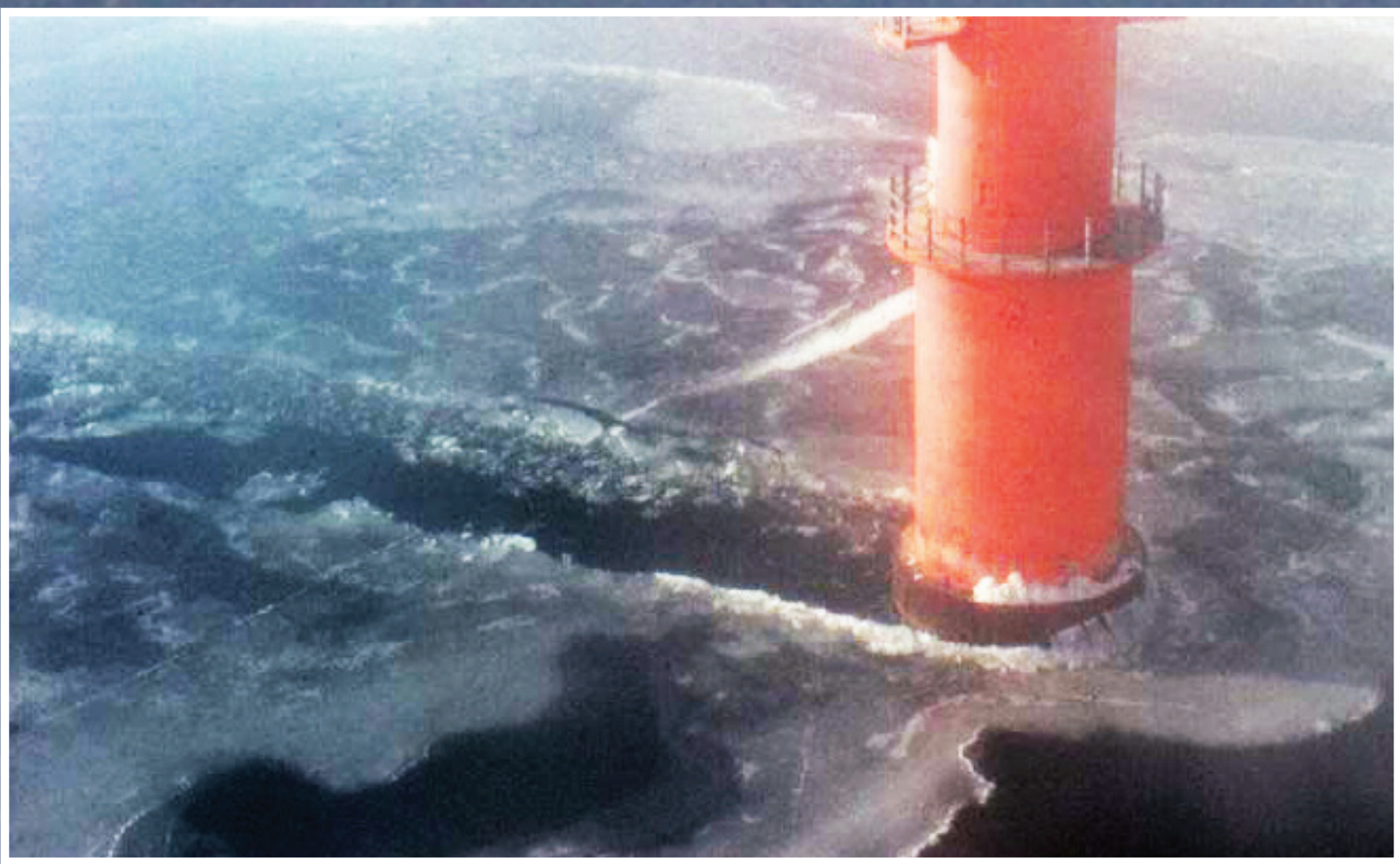
Low ice load from drifting ice against a lighthouse.
