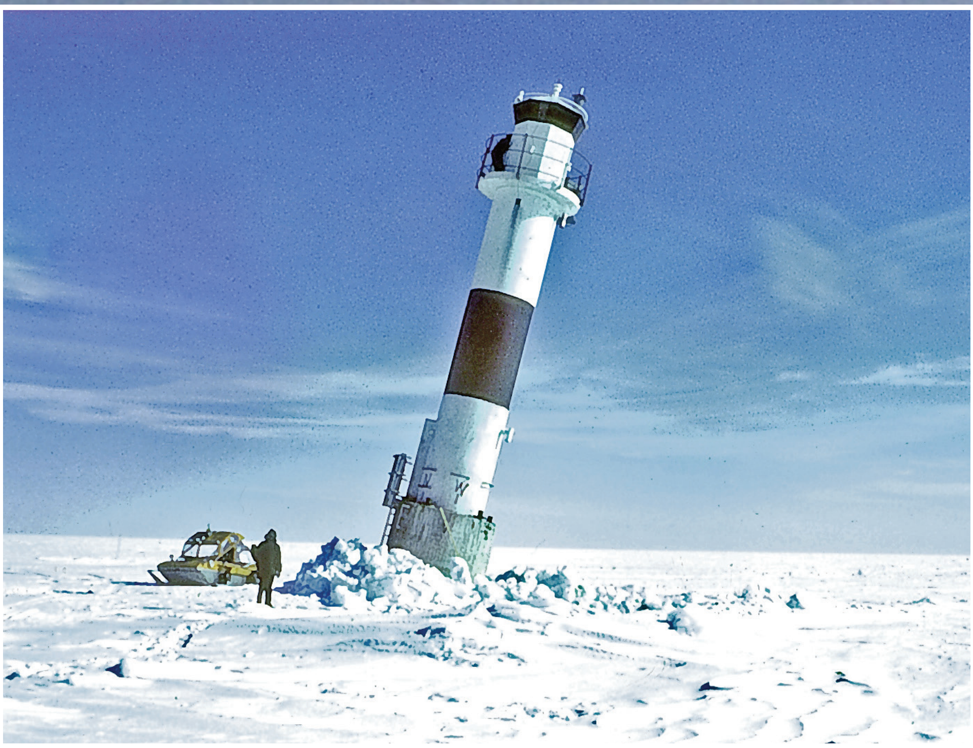
Björnklack, April 1985. The lighthouse in the Bothnian Bay was subjected to extreme ice forces. It was displaced 17 meters and tilted 12 degrees. The ice load was estimated accurately to 1090 tonnes!
