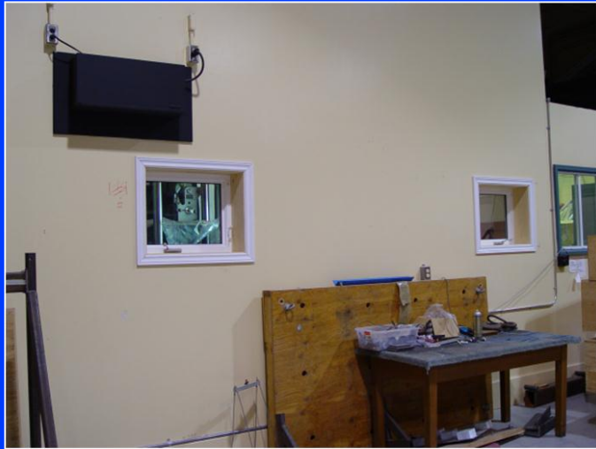
OCRE/NRC Cold Room with Windows
