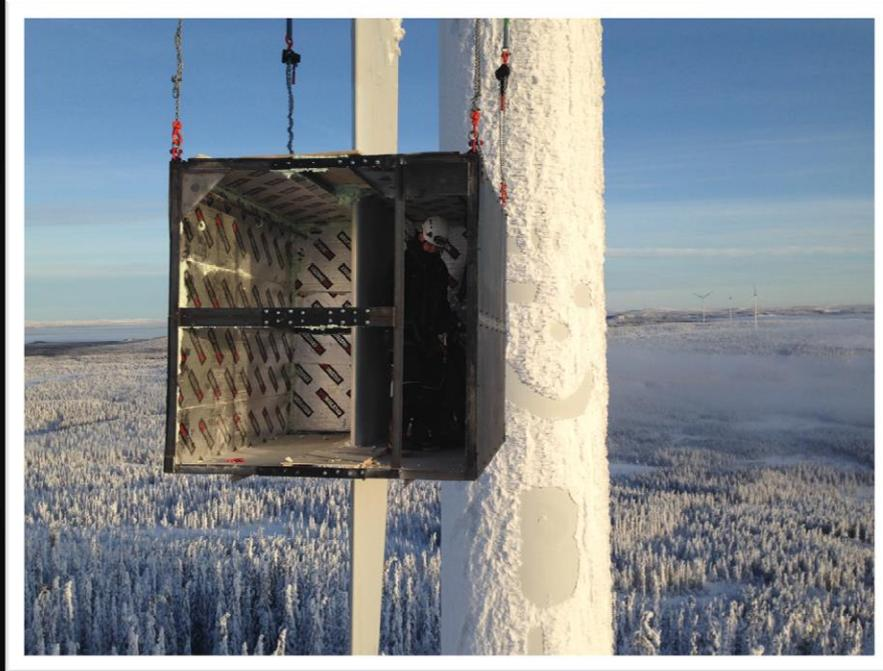
Blade repair module provided safe and stable working conditions for repairs
