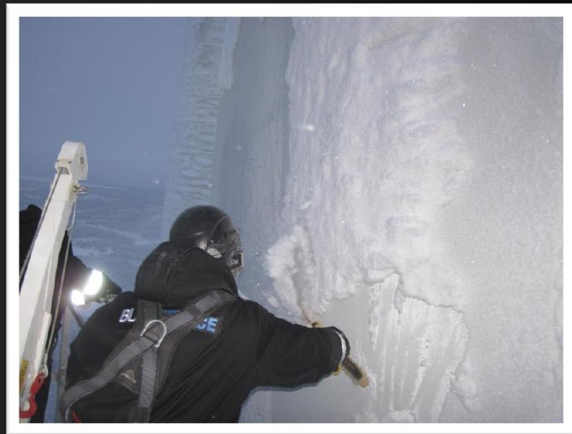
Prior to work ice was manually removed from the blade
