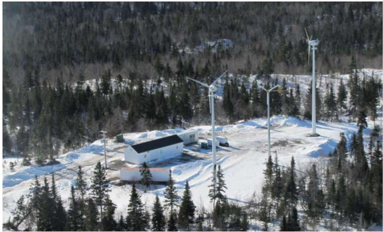
57, 5 kW wind 100 kW diesel 5kW solar AC & DC buses Off-grid
