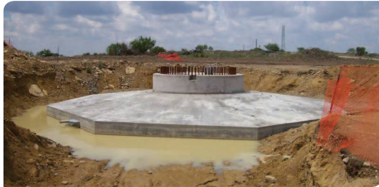
Figure 2. Example of gravity foundation under construction.
