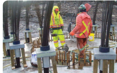
Figure 3. Example of rock anchored foundation under construction.
