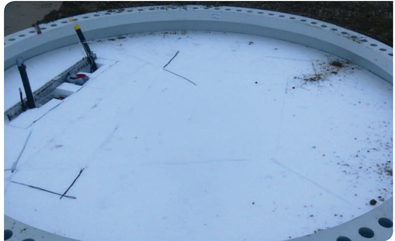
Figure 15. Insulated wind power foundation.
