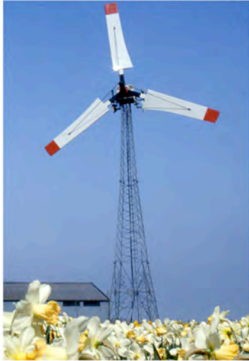
Grid connected turbines; small scale
