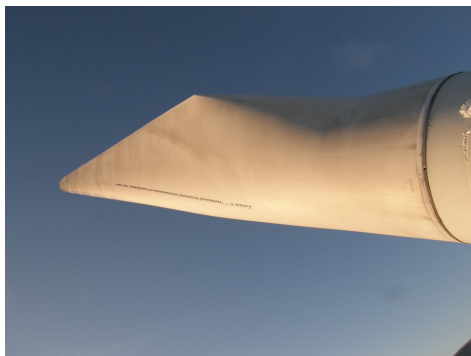
Turbine 3 - Ice prevention in operation
