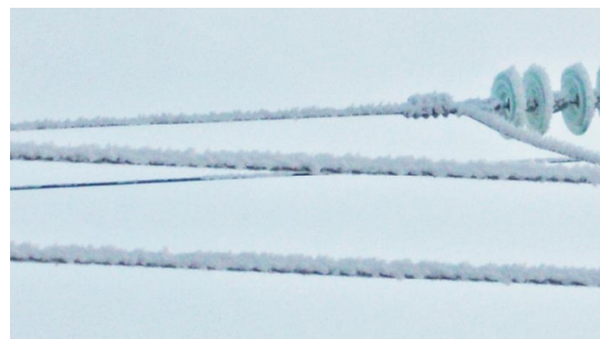
Figure 7. Frost formation on wire lines “Bugulma-110–Karabash” December 1, 2014 at 10 o'clock 16 minutes, which corresponded \delta K = 0.3 dB/km and \delta\tau = 0.1 \mu s/km (snapping time is marked in Figure 5 with cross)
