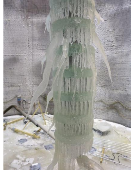
Figure 10: Close view of the insulator covered by glazed ice accreted under full DC voltage 361 kV. Note long icicles developed along the E-field lines.
