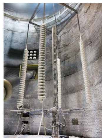
Figure 2: Final set-up for four insulators in parallel during ice accretion without voltage (rime ice).
