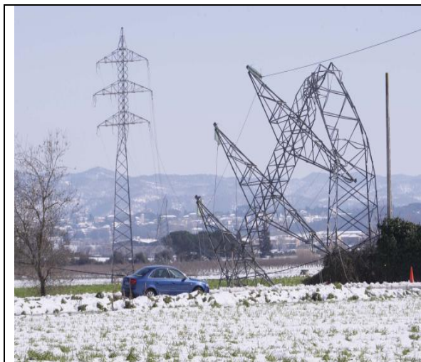
Fig 04 : Tower line 110kv, 2 circuit , bent by the combined action of wind and snow
