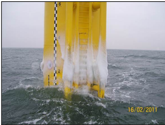
Figure 7: Ice-covered leg of wind turbine platform in the Baltic Sea
