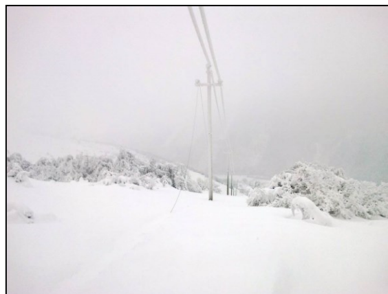
Figure 1: broken MV conductor on ground due to strong wet-snowfall event in central part of Italy.
