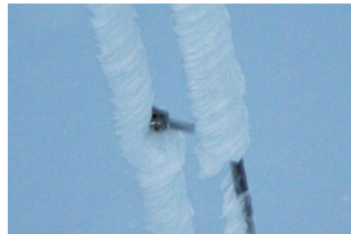
Fig. 11. In-cloud icing on duplex conductor in FL4 (400 kV OHTL) in Dec. 2006.
