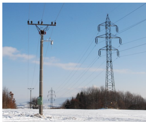
Figure 1: Monitoring station PMS installed on MV line
