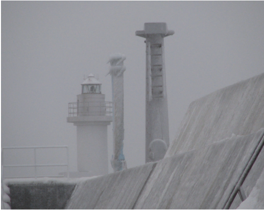
Figure 3: Dummy light beacons on breakwater at Hamamasu Harbor. Stormy weather often generated not only heavy spray jets but intense snowfall.
