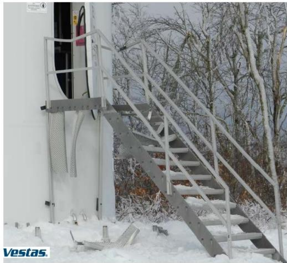
Figure 19: Damaged stairs from an ice fall
