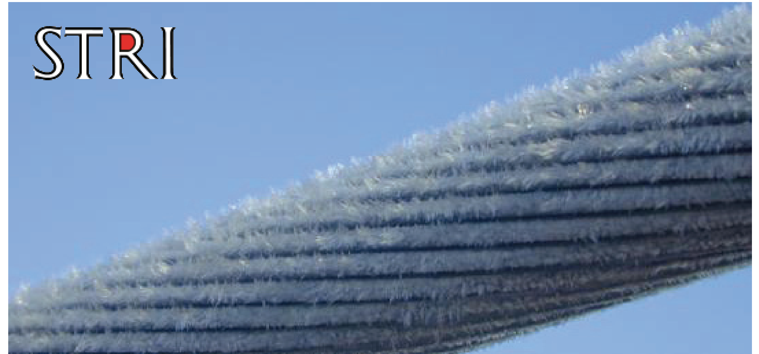
Example of hoar frost on a conductor
