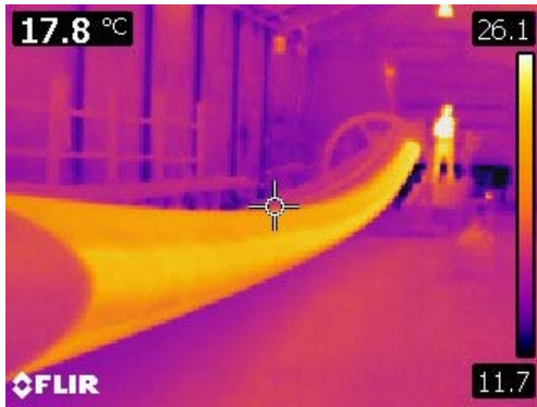
Test the system at the plant
