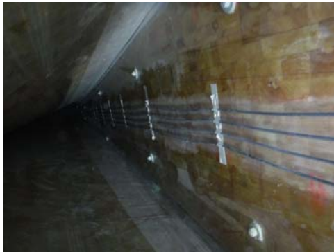
Cables and heating mat installation
