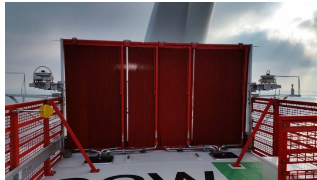
heating / cooling systems
