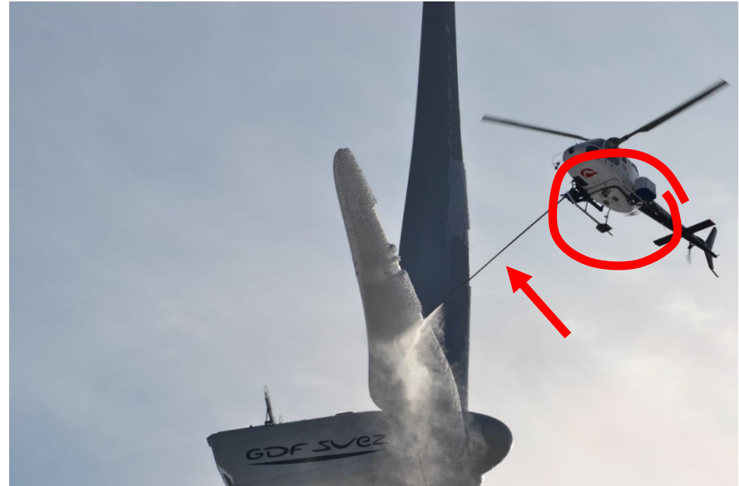
De icing (Vestas V90) with hot water and a helicopter in Canada
