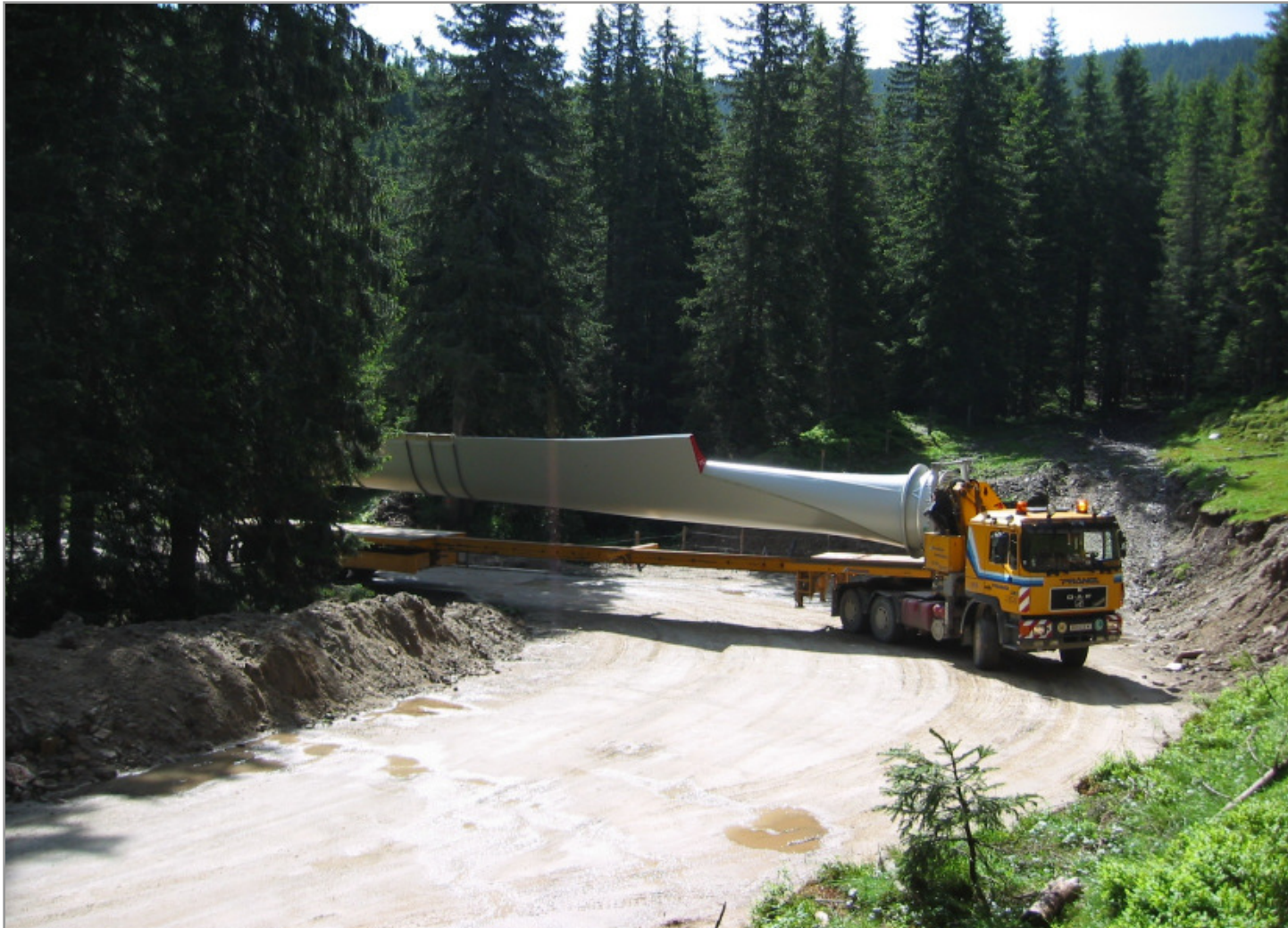
Construction of Wind Farm Moschkogel
