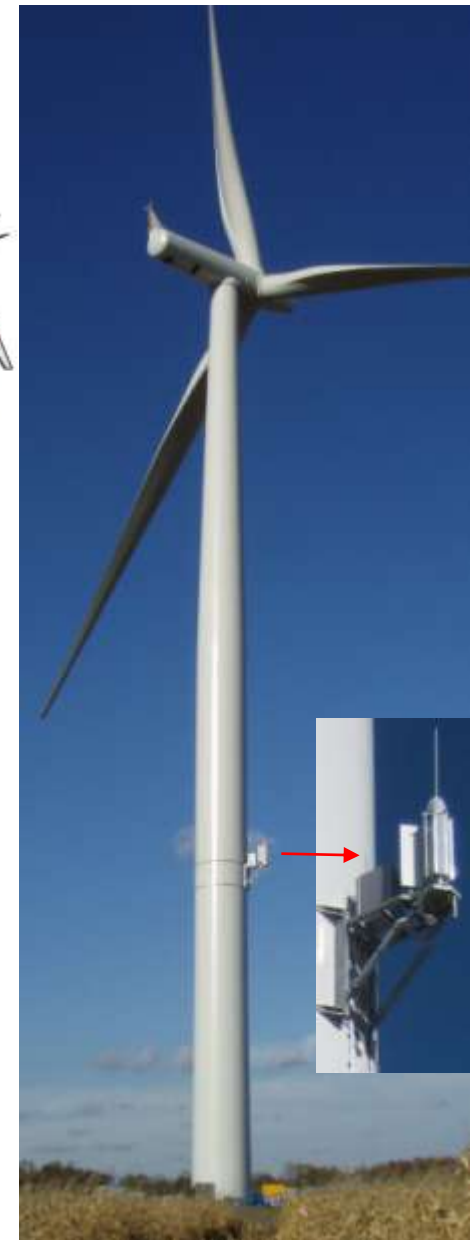
OCAS radar at Siemens SWT 2.3-101 in Ontario, Canada (Talbot wind park)
