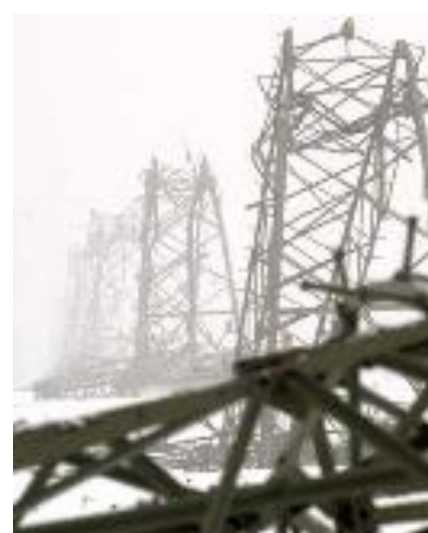
Fig. 3: Damaged power line poles in Münsterland area on 26.11.2005 (Photo © DPA, 2005; see [2] and [3] for more information)
