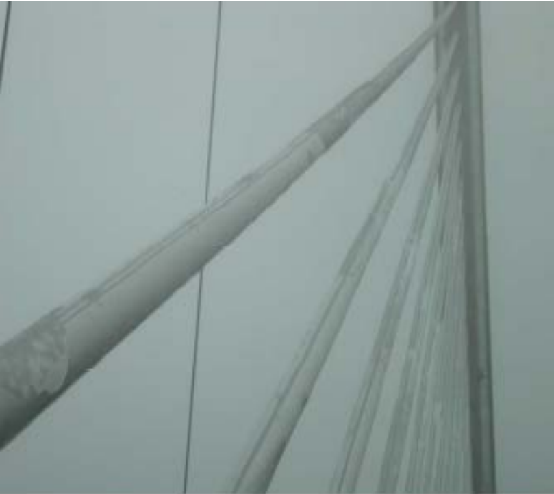
Ice accumulation pattern on VGCS stays
