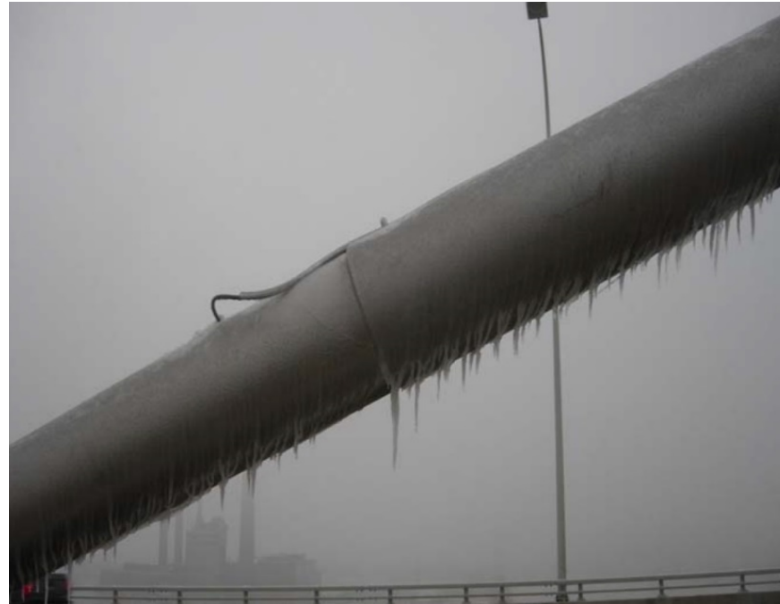
Ice accumulation on the east side of VGCS
