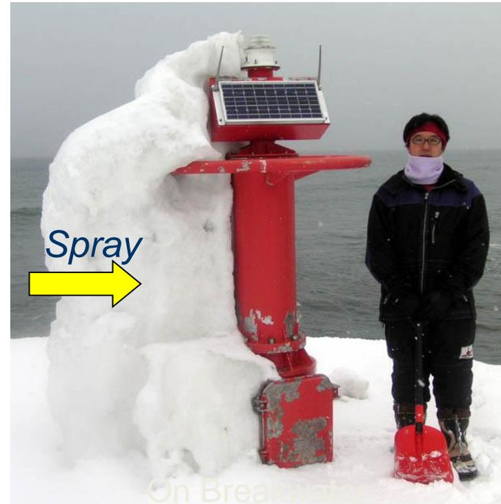
Freezing spray is the main cause of spray icing.
