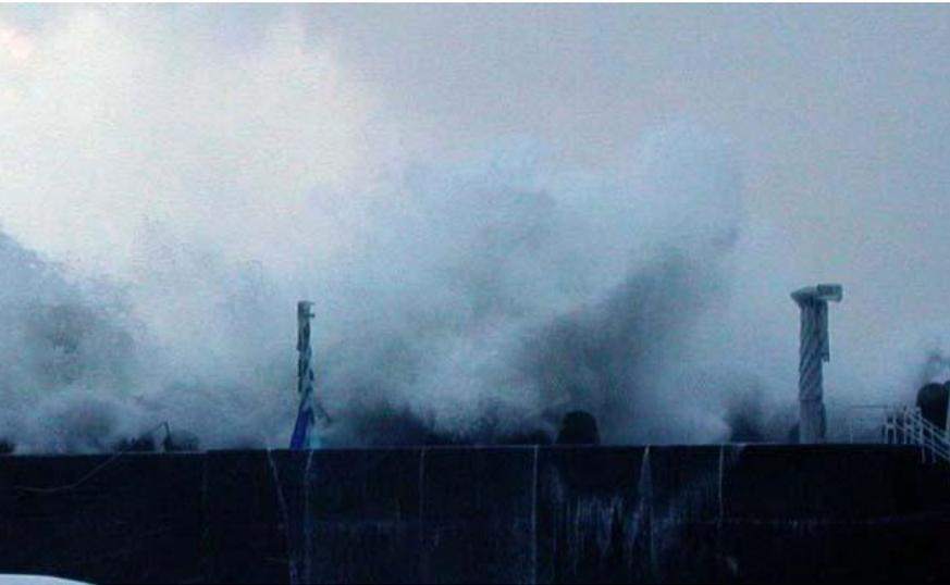
High waves caused by north-westerly wind often generated a heavy spray jet at the dummy light beacons. The spray icing grew under heavy sea-water spray and during low temperatures.
