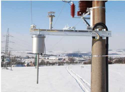
Figure 2: Support arm with sensors
